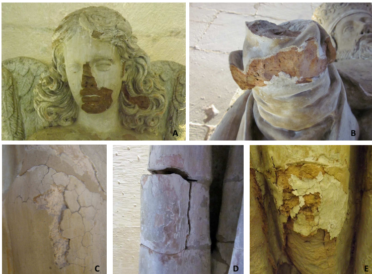
Fig. 5 – A) Loss of material by dustiness; B) Loss of a hand; C) Craquelures; D) Fractures; E) Flaking
